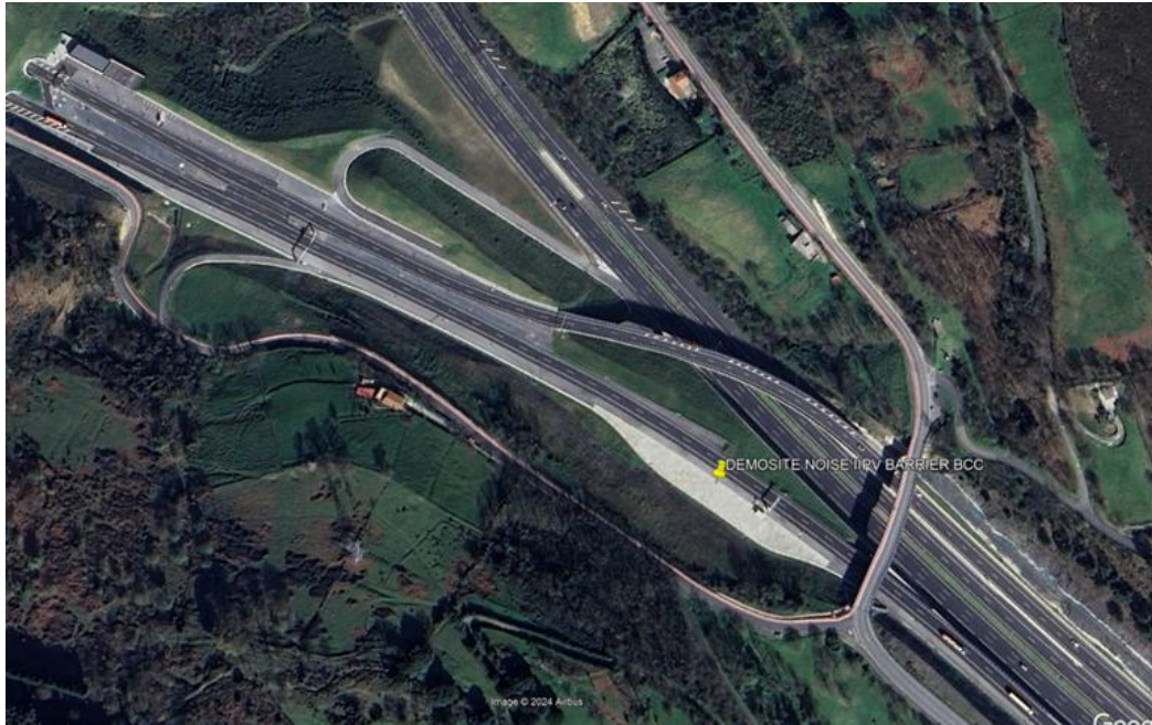
Figure 2.18: Demo 6 – Aerial view situation
