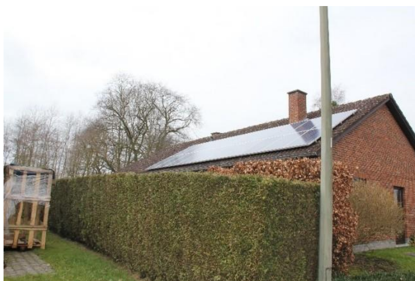
Figure 2.10: Demo 4 – Picture of the demo building
