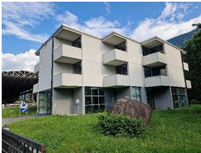
Figure 2.7: Demo 3 – Picture of the building
