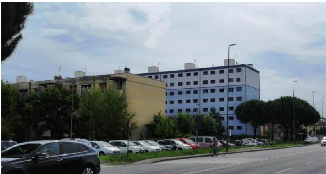
Figure 2.1: Demo 1 – Picture of the building
