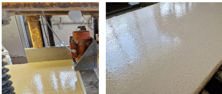
Figure 2. Mortar finishing after power screed resetting
