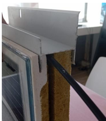
Figure 2-16: Aluminium H-profile placed inside the upper horizontal grooves
