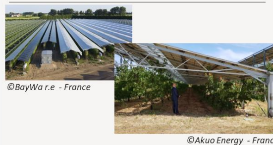
Elevated PV without tracking
