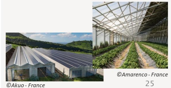
PV integrated in greenhouses
