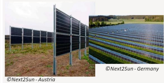
Vertical bi-facial PV with grazing or agricultural activity in interspace
