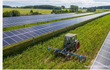
Ground-mounted PV with agricultural activity in interspace
